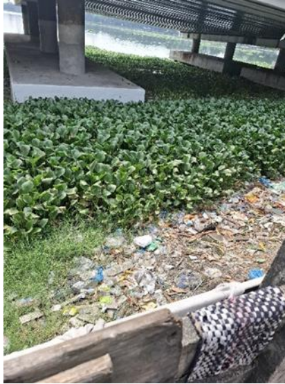
Figure 1.2. Retention Pond ( Bozem ) in the Morokrebang Area, Krembangan, Surabaya
